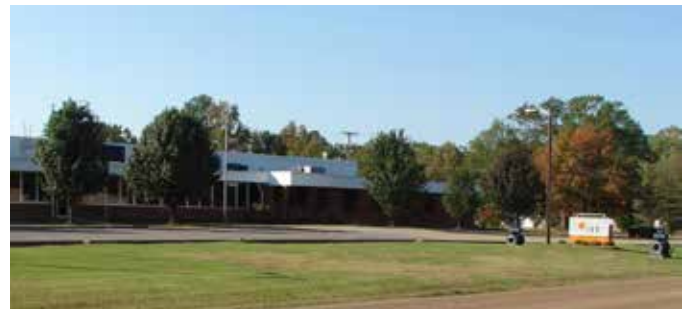
Amory, MS Facility
