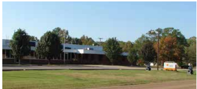
Amory, MS Facility
