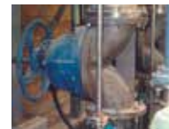
Massachusetts Config: Dia-Flo Weir Size: 8"
