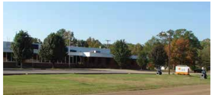
Amory, MS Facility
