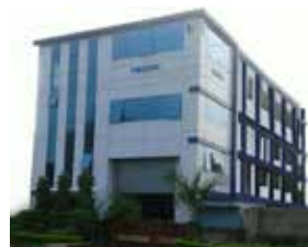
Tecnik Fluid Controls Pvt. Ltd. Mumbai, India
