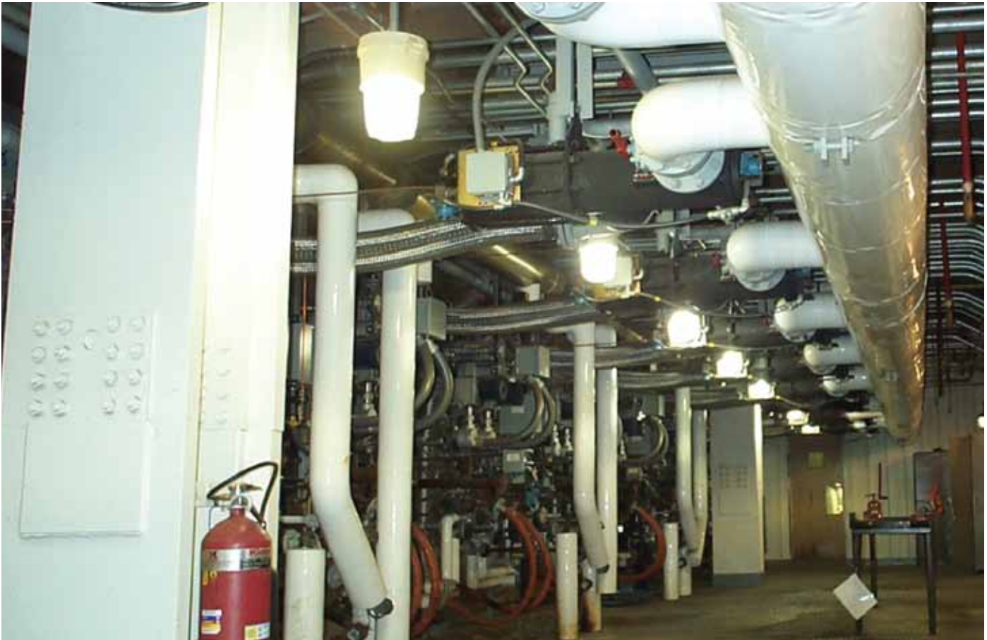
T4600F (6 inch) Skotch Trifecta gas valves are installed above the burner level in the horizontal position, which reduces burner front clutter.
