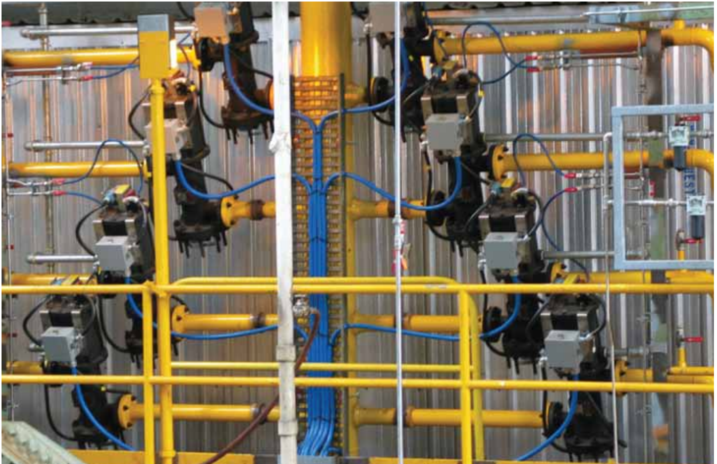
Shown are eight T4300F (3 inch) Skotch Trifecta gas valve systems replacing the need for twenty-four independently actuated valves. Installation time and space are reduced considerably.
