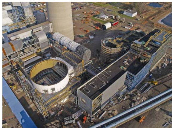
Construction of the WFGD system at DP&L's Killen Unit
