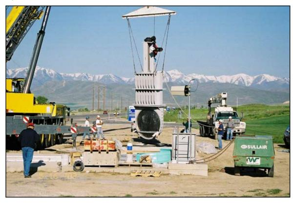
ITT EV offers bonneted Fabri-Valve knife gate valves for difficult services such as buried service requiring gate protection and high cycle stem sealing. The cylindrical packing around the stem provides a tight, easy to maintain stem seal. The 72" valves used in this aqueduct had:
