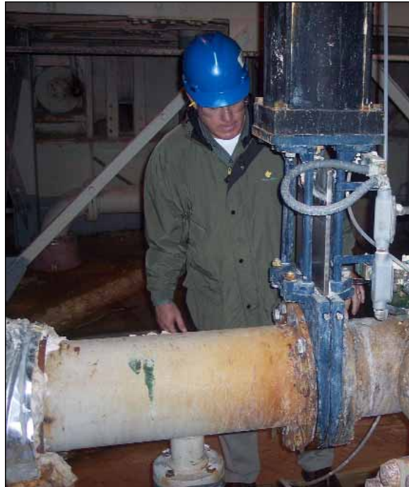
A 10" actuated knife-gate valve (Model XS150-ULV) from ITT on a gypsum slurry line for FGD service.
