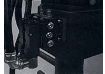
Existing Valve Configuration
