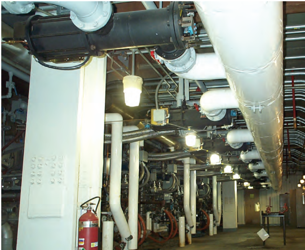
T4600F (6 inch) Scotch Trifecta gas valves are installed above the burner level in the horizontal position which reduces burner front clutter.
